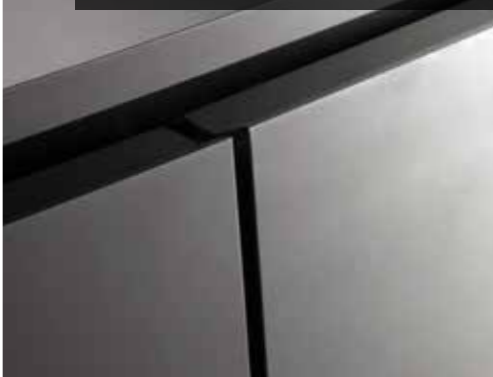
V-cut for all visible bendings
